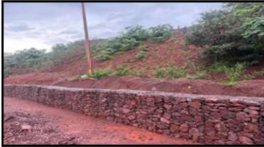
Retaining wall & Garland drain
