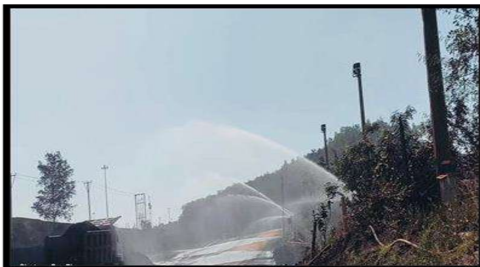
Fixed Water Sprinkler
